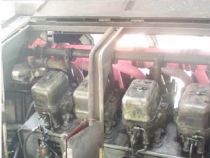
Notch 8 during loadbox test: exhaust gas manifold is red-glowing
