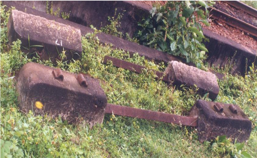
RCC SPLIT SLEEPER WITH TIE BAR
