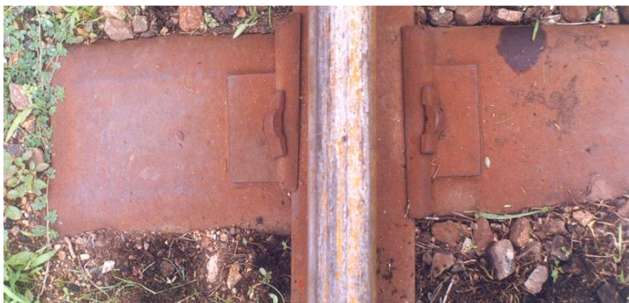
S T SLEEPER WITH FIXED JAWS
