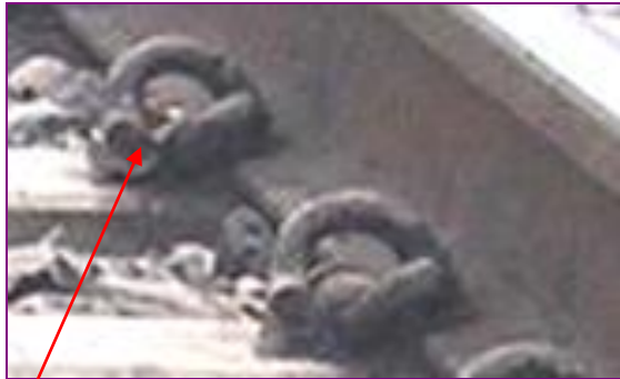
Pandrol clip (or) Elastic rail clip
