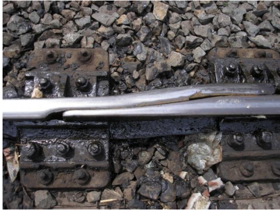
Switch expansion joint (SEJ)
