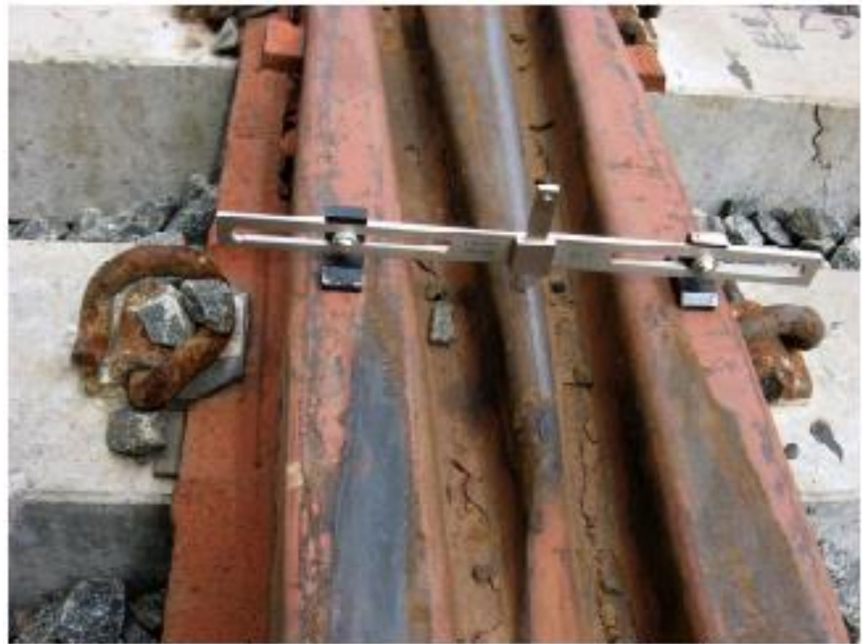
Measuring the wear at the nose of the rail
