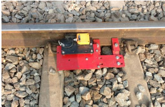
Proximity Sensor fitted inside the track
