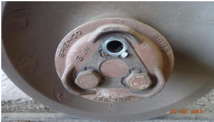
Fig. 9: Missing Cap Screw
