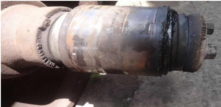
Fig.15: Cocked Grease Seal
