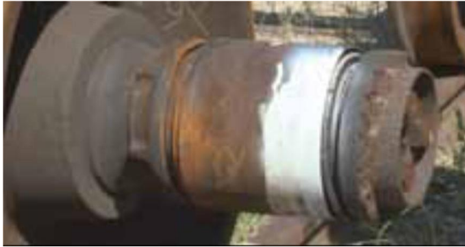
Fig. 8: Phenomenon of discoloration due to overheating
