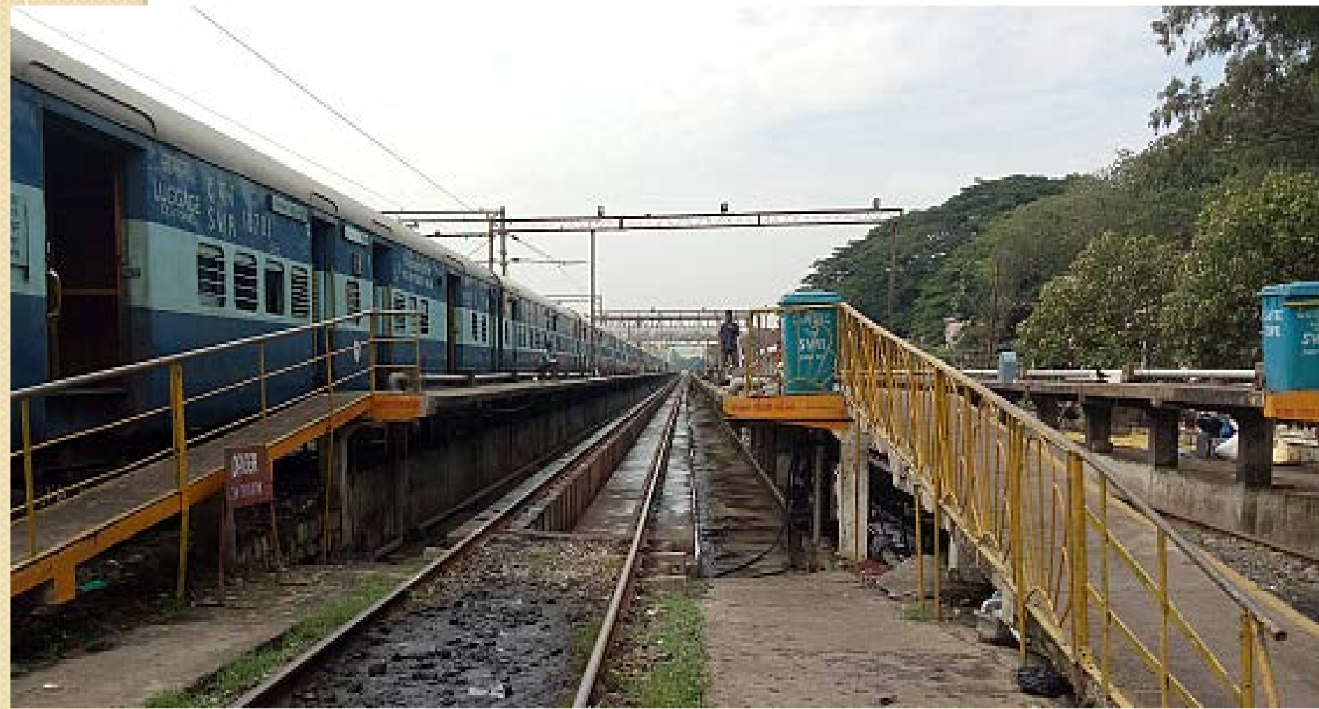
Pitlines: 5 & 6 (with catwalk)
