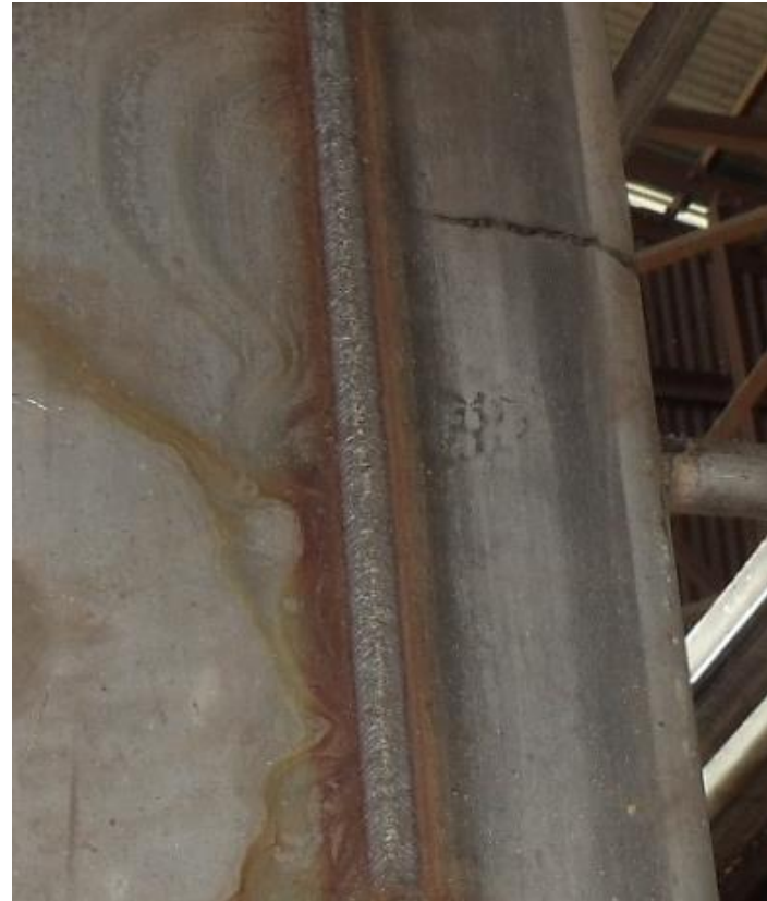
V. Welding with aid
