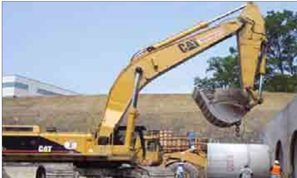
Excavator in action
