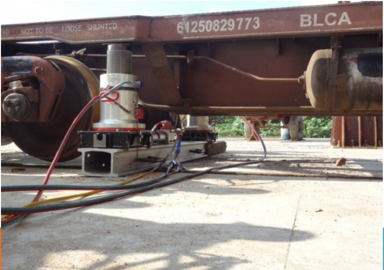
Hydraulic Rerailing Equipment in Action
