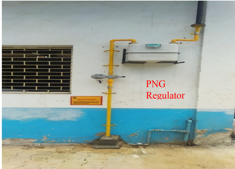
PNG pipe line and regulator at Mechanized laundry Gwalior
