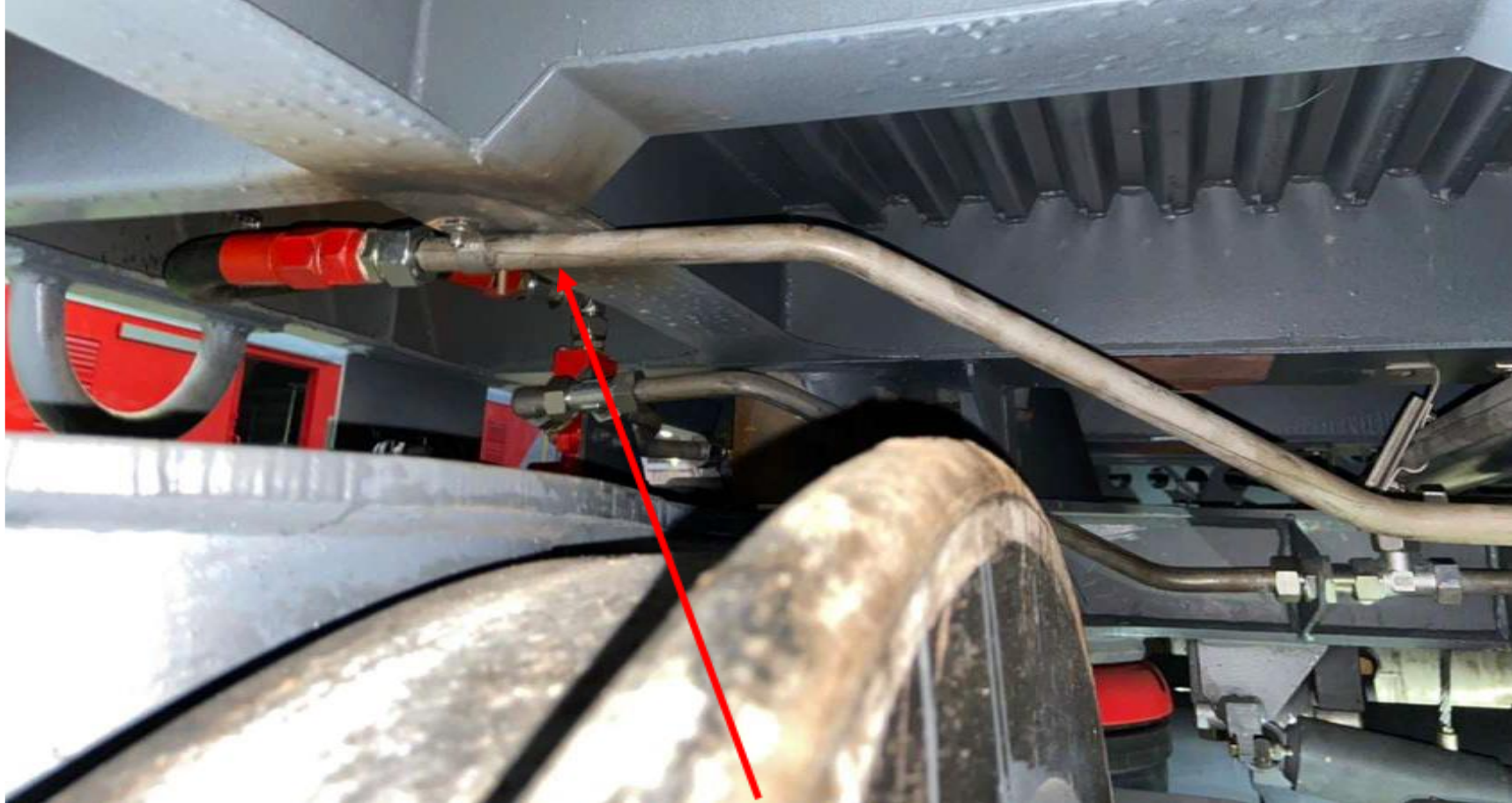
CLOSER VIEW OF SHIFTED STEEL PIPE TOWARDS COACH END
