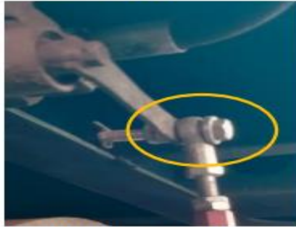
Cause no.02 -Incorrect Fitment of washer, bolt & levelling valve horizontal lever etc.
