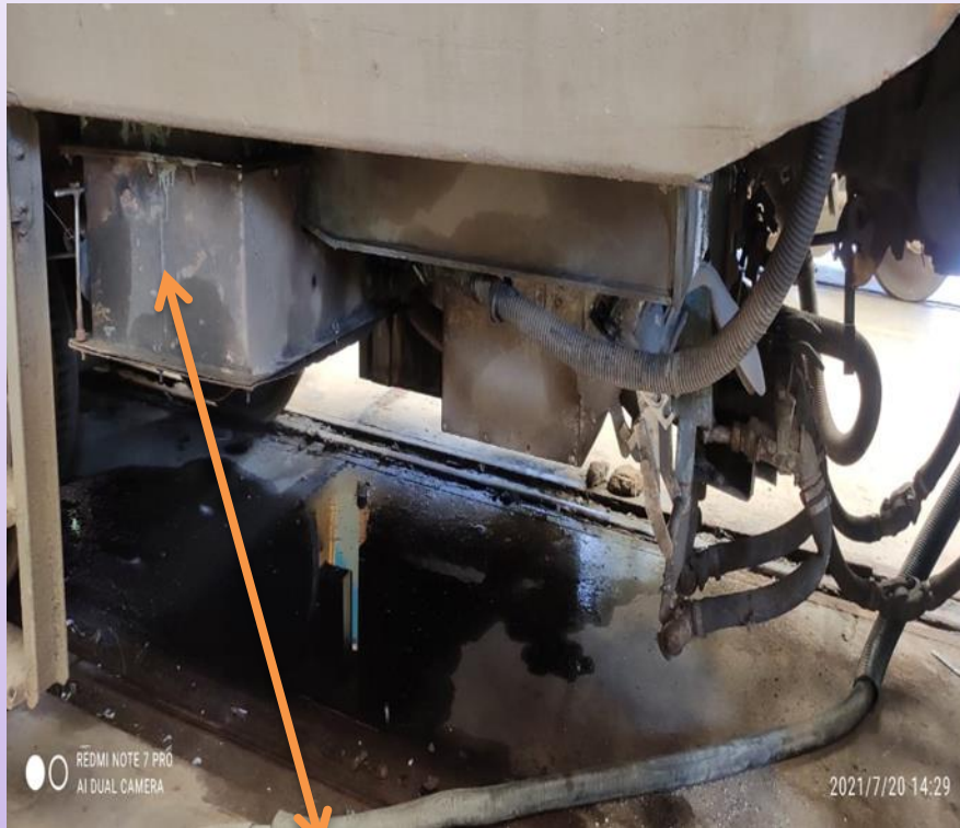
INSPECTION BOX under AC panel
