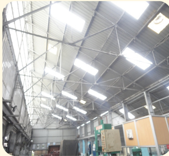
Provision Of Transparent Roof Sheet In Shop Floor
