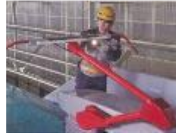
Inspection of Pantographs / Replacement of contact strips
