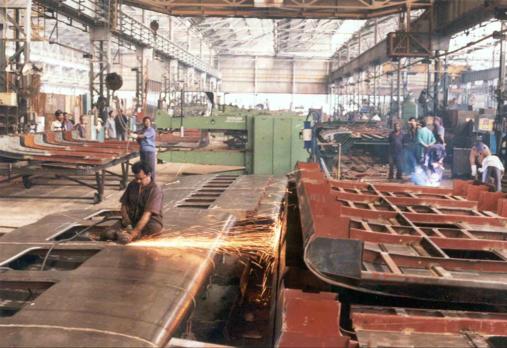
FINISHING OF SIDE WALL
