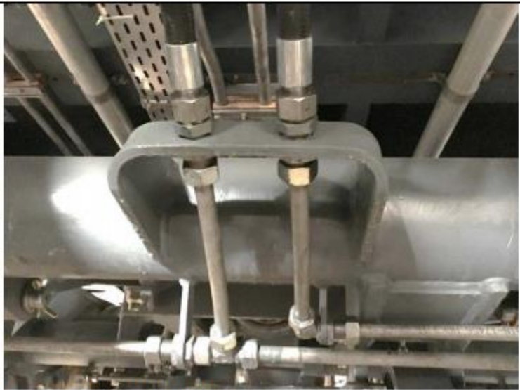
Modified piping arrangement with reduced joints and modified hose
