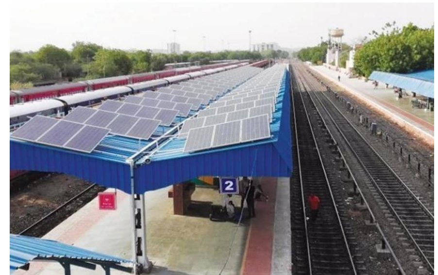
Asangaon Railway station of Central Railway under Mumbai Division has been declared 100% Green Powered Station in March, 2018 as it is powered with windmill and solarpanels
