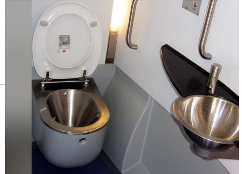
Bio-vacuum toilet in train
