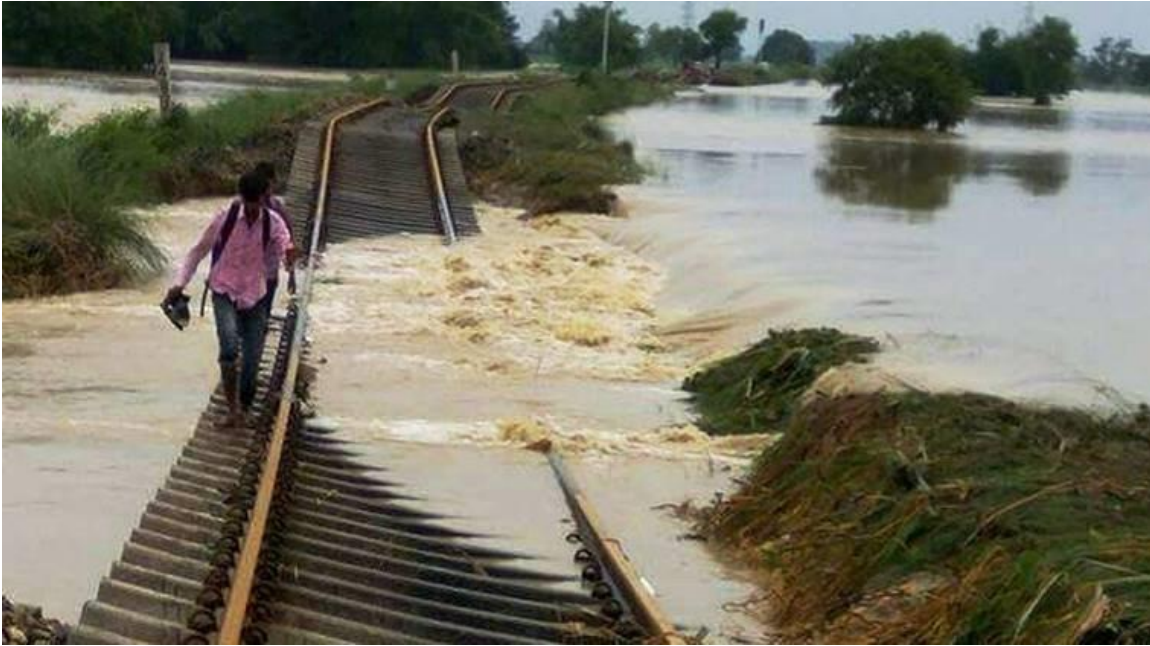
Damaged railway line in flood-hit Katihar district (August 2017)
