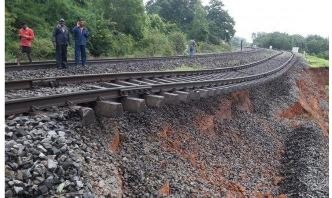
Soil bed under the track washed off due to heavy rain in Uttara Kannada (August 2019)
