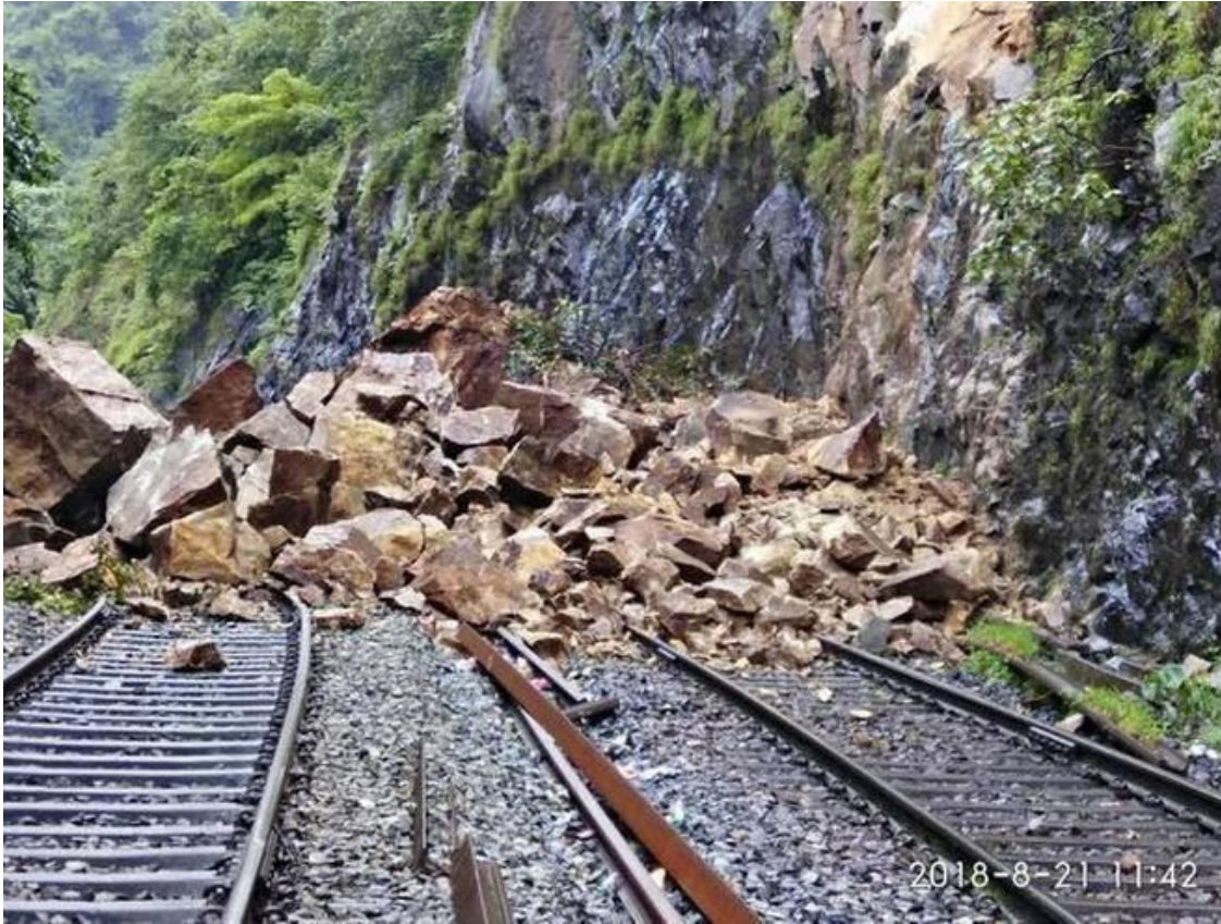
Landslide on the railway track on the Karnataka-Goa border (August 2018)
