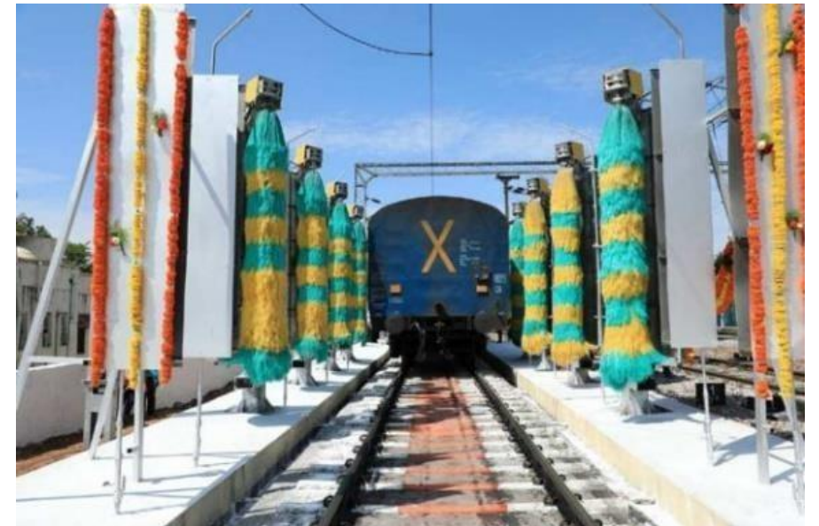
12 Automatic Coach Washing Plants have been installed in 2018-19
