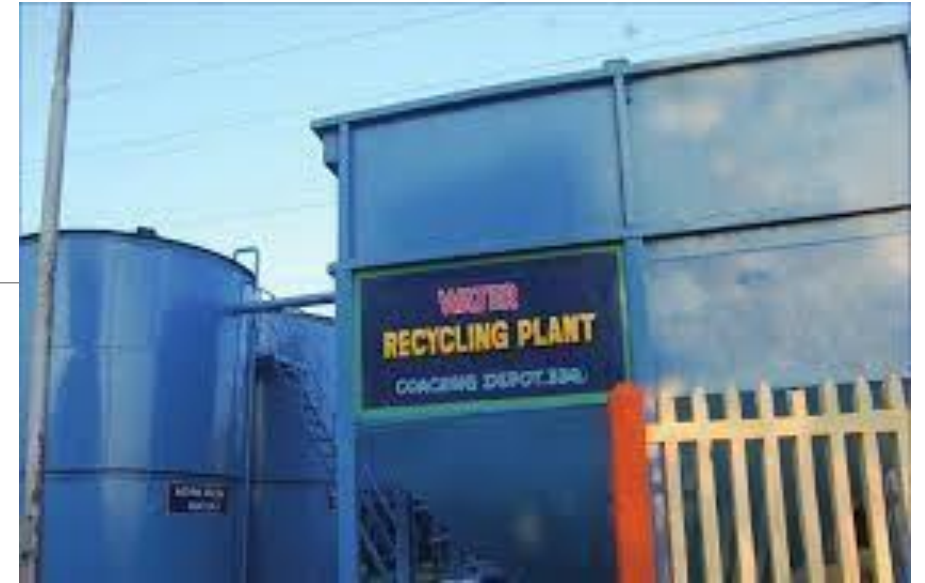
Water recycling plant at Indian Railways Coaching Depot
