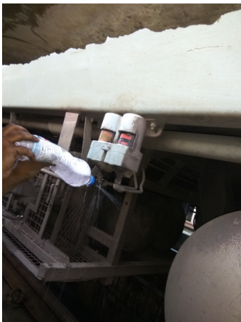
Check for air leakages at joints by means of soap solution
