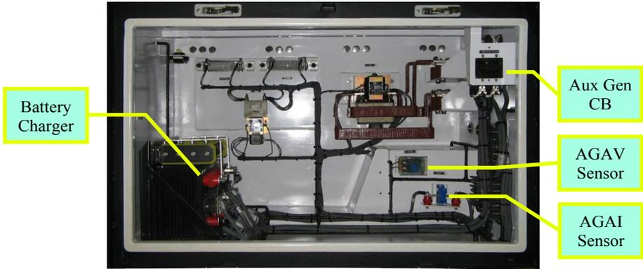
Fig. 5.3 Internal View of ECC#2
