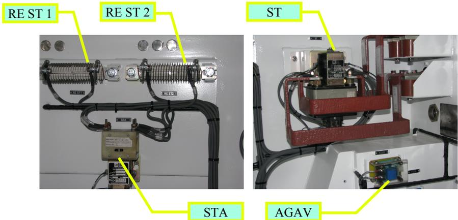
Fig. 5.4 ST Contactors and Resistors in ECC#2
