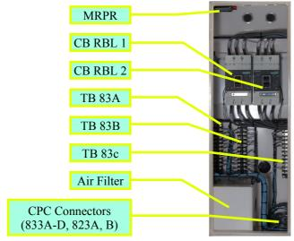
Fig. 5.7 Fan Contactors in ECC#3
