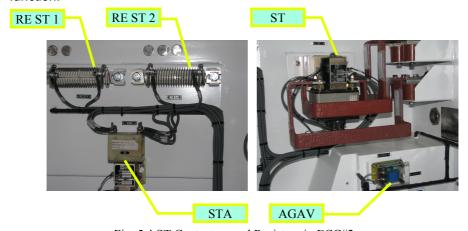
Fig. 5.4 ST Contactors and Resistors in ECC#2
