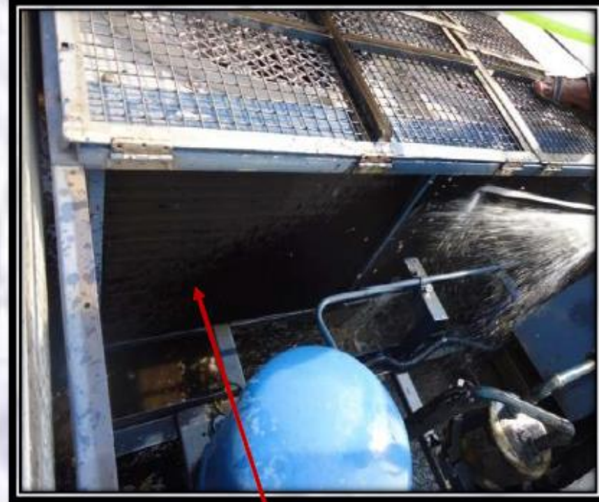
Condensator coil after cleaning
