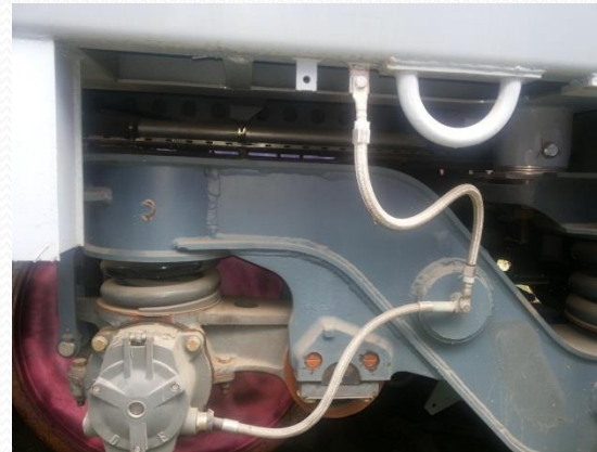
Shell body to bogie frame earthing cable
