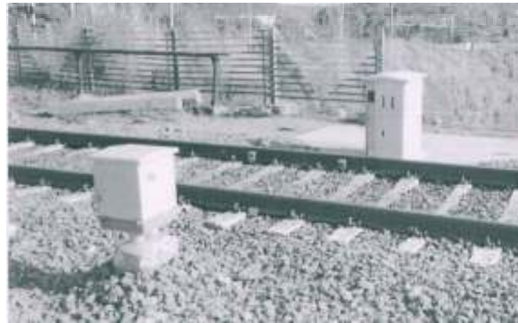
Hot Box detector for hot bearing
