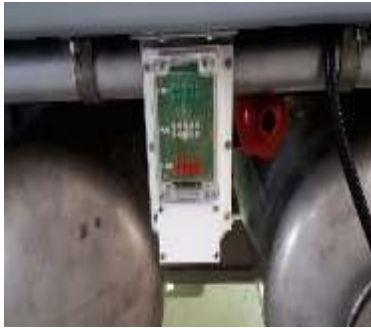
Water level indicator fitted near water tank
