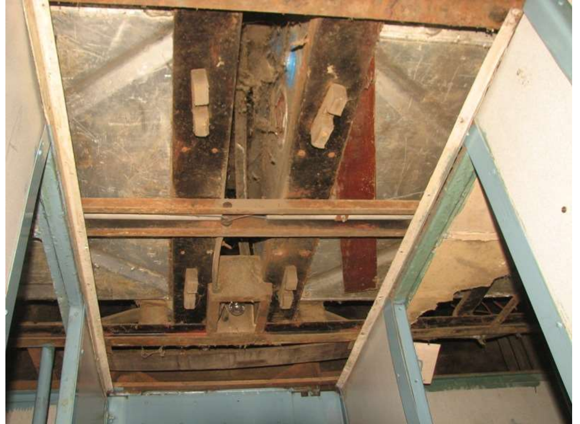
Coach Water Tank Area
