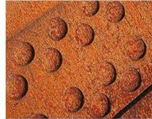
Rusted Riveted Steam Engine Boiler
