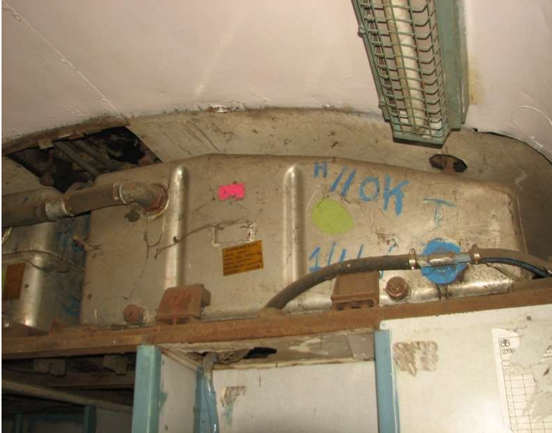
Coach Water Tank area
