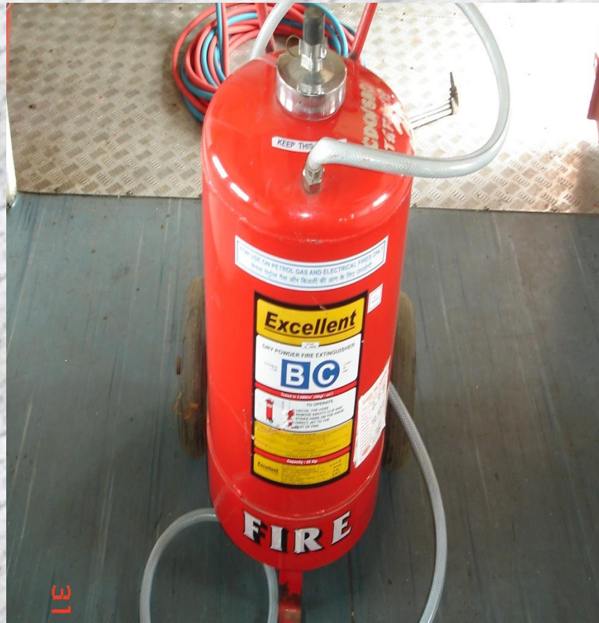
25 Kg capacity DCP Fire Extinguisher
