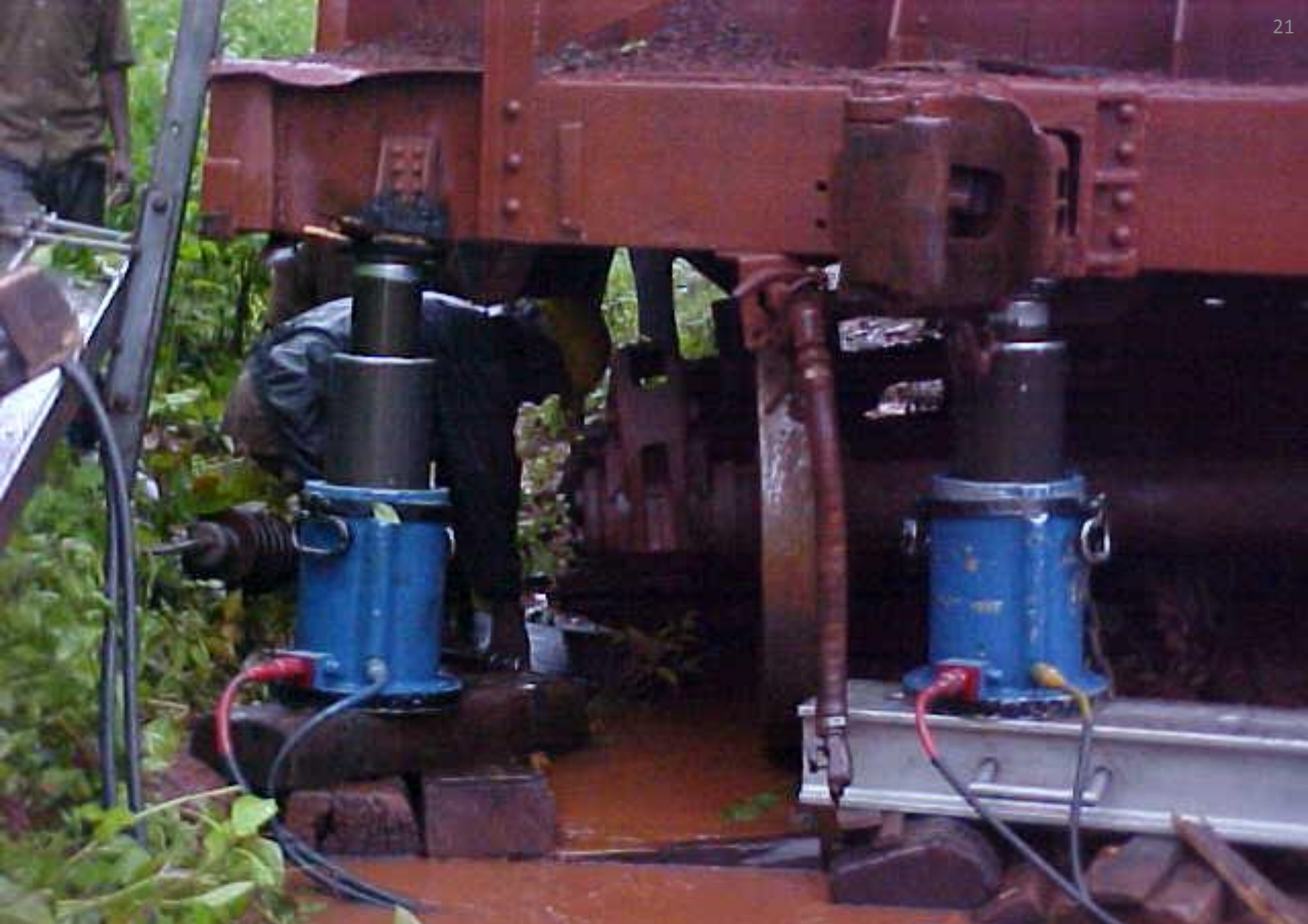
Lifting by Hydraulic Jacks in water logging & raining condition to re-rail BOBS (L) on 12.08.07
