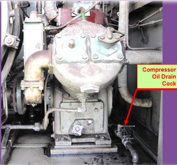
Fig. 1.61 Compressor Oil Drain Cock
