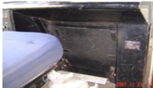
Open cover below the controller
