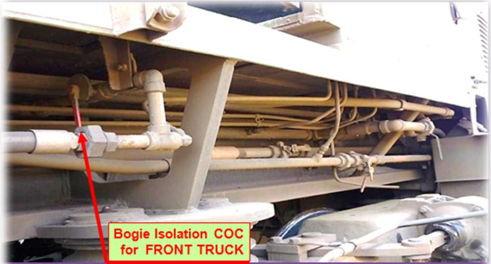
Fig. 1.48 Bogie Isolation COC for Front Truck
